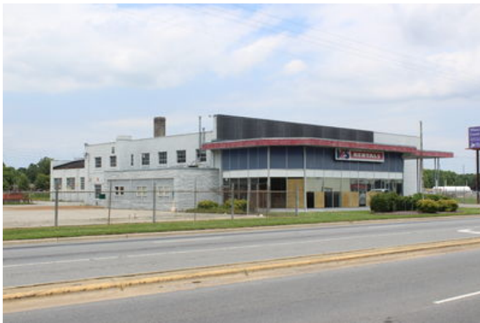
22,497 +/- SF Industrial Building
