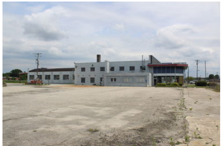
Side of Building
